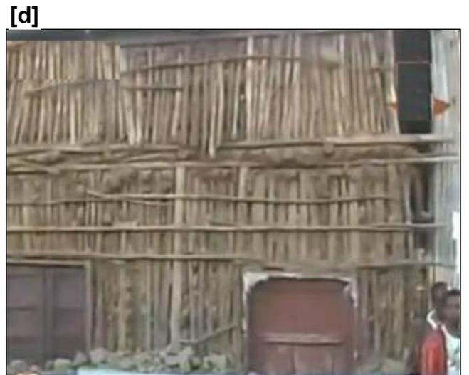
**Figure 6.** Photographs of structural damages due to the December 2010 Hossana earthquake. [a]-[c] show damages to reinforced concrete frame dormitory buildings at Jimma university where 26 students were injured. [b] structural damage to slab and column joint. [c] debris from damaged frame. [d] damage to the masonry clad of a timber building. EBCS-8:1995 classifies Jimma as seismic zone 1. Image Source: Ethiopian TV.
